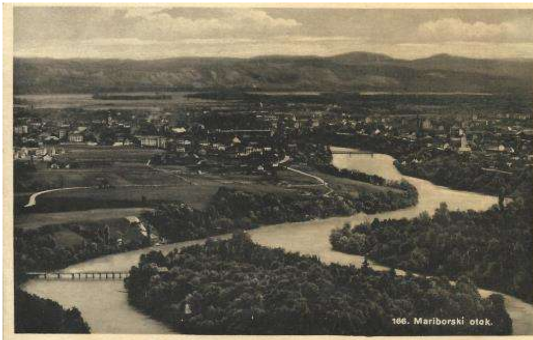
Slika 40: Leseni most in otok (Vir: Stanka in Božidar Damjan 1995)
