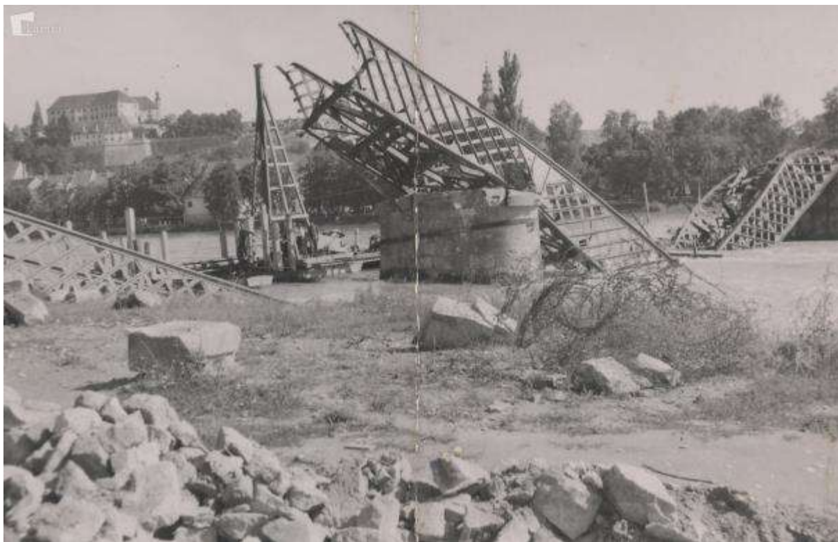
Slika 116: Porušen most (Vir: www.kamra.si/digitalne-zbirke/item/zelezniski-most-1860 )
