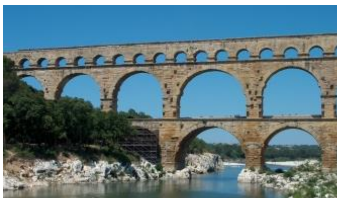
Slika 4: Akvadukt [Vir: http://cdn.history.com/sites/2/2015/03/history-lists-10-innovations-that-built-ancient-rome-aqueducts_Corbis-A.jpeg , 9.2.2016]
